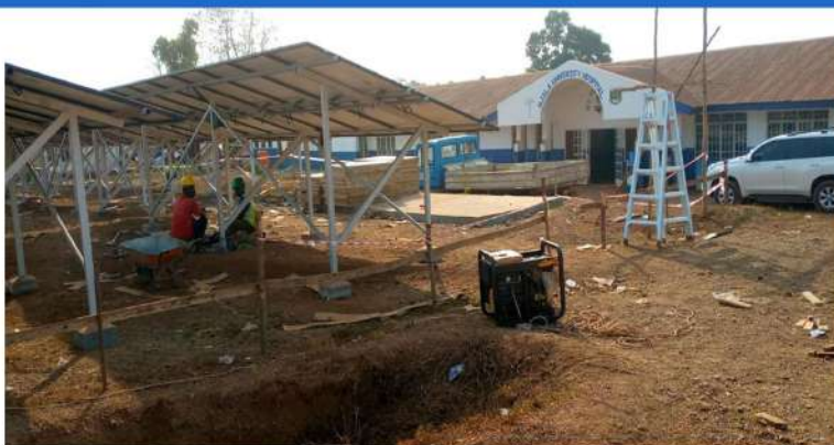
Solar panels installed to generate and distribute electricity to Njala University Hospital
